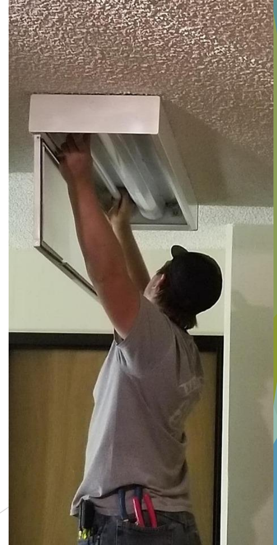
LIGHTING UPGRADED TO LEDS
