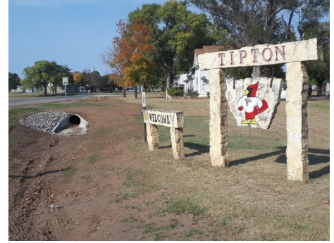
A recent project in the City of Tipton improved the city's storm drainage system.
