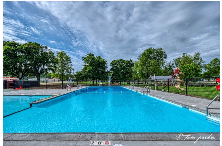
The City of Blue Rapids swimming pool project was completed earlier this year. (Photo courtesy of Tom Parker)
