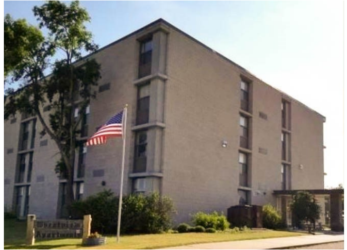
An example of a recent multi-family weatherization project that NCRPC administered in Ness City. The NCRPC administers the Weatherization Assistance Program for 41 counties in Kansas.
