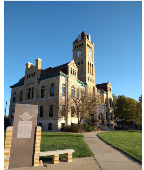
Mitchell County utilized the State Historic Rehabilitation Tax Credit Program for an exterior restoration project on its courthouse this year. (Photo courtesy of Doug McKinney)
